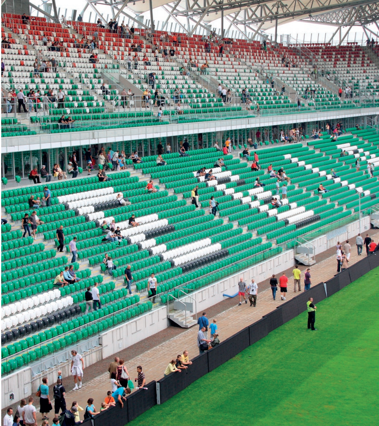
The Marshal Józef Piłsudski Legia Warsaw Municipal Stadium, Warsaw
