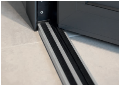
Aluminium threshold with a thermal break
